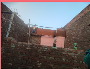
Flood Relief Housing Reconstruction
